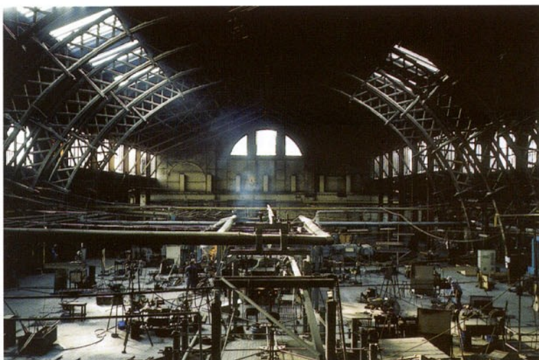
An architectural landmark – the production hall of Glashütte Lamberts with its beamed and filigreed roof construction. Originally designed in the 19 th century as an agricultural exhibit in Nurnberg, the building was moved to Waldsassen in 1907.
